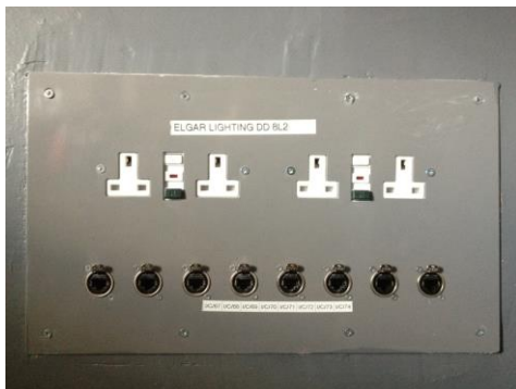
Network points and 13 amp sockets
